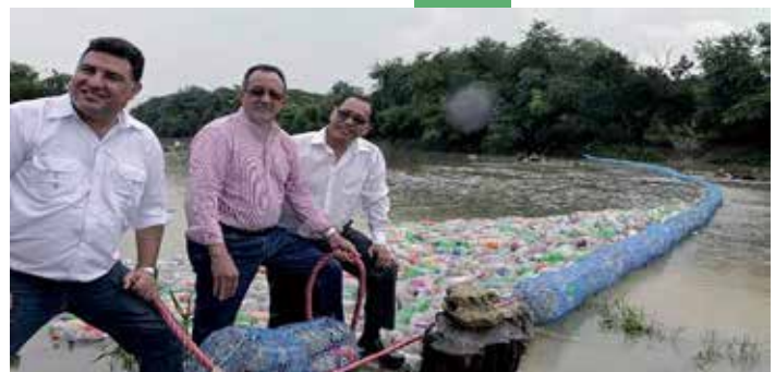
► Photo: Ministry of the Environment and Natural Resources, Dominican Republic Installation of biobardas (floating biofences) in Dominican Republic.
